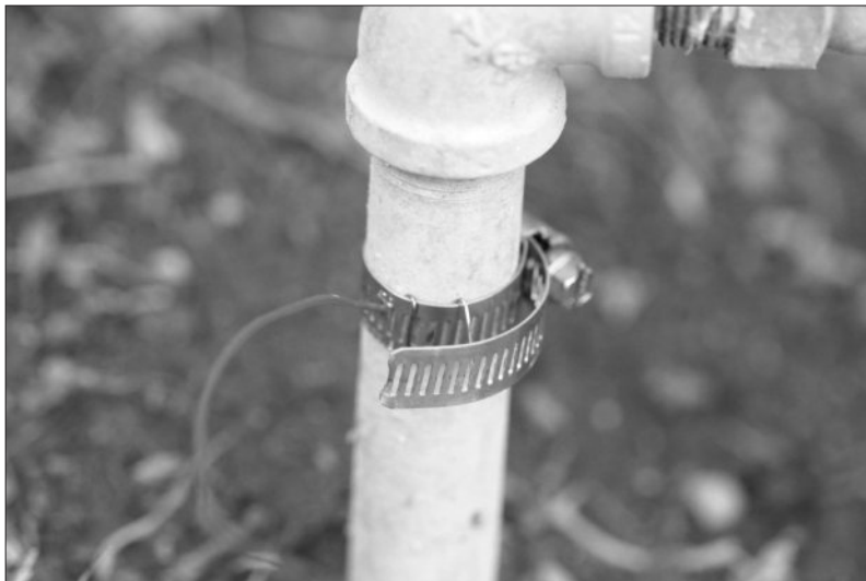
Figure 2-6: A good ground connection.
