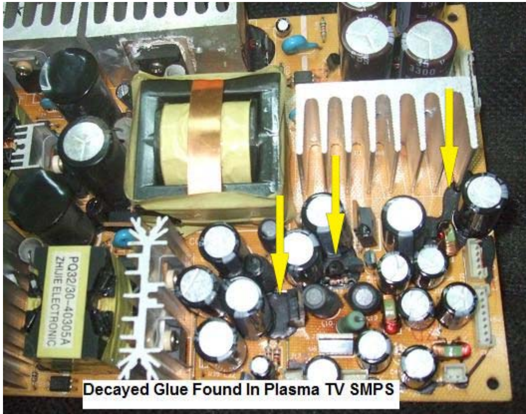
Figure 15.12- Decayed Glue Found In Circuit Board
