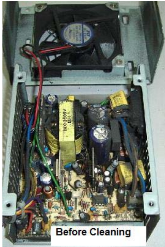
Figure 20.6- Dirt Inside The Power Supply
